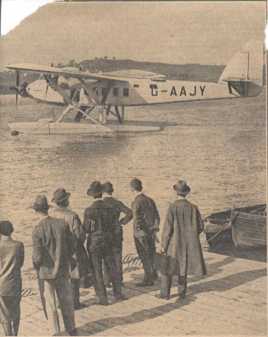
SEAPLANE TEST.—Claimed to be the biggest seaplane, the Valetta, constructed by Messrs. Short Bros., was tested at Rochester yesterday. It has three Bristol Jupiter XI F engines and has a cruising speed of 120 miles an hour.
